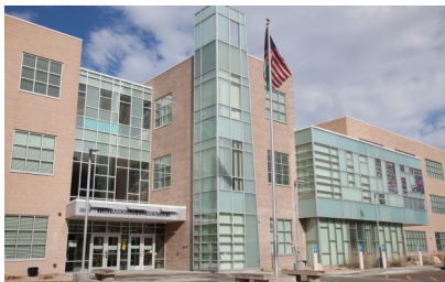
Timpanogos Elementary (K-6) Year Rebuilt: 2008
