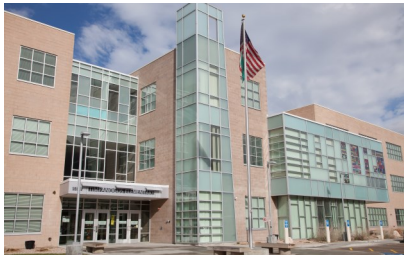
Timpanogos Elementary (K-6) Year Rebuilt: 2008
