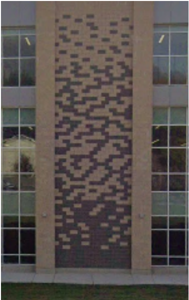
Decorative brick panels to be replaced with standard painted brick
