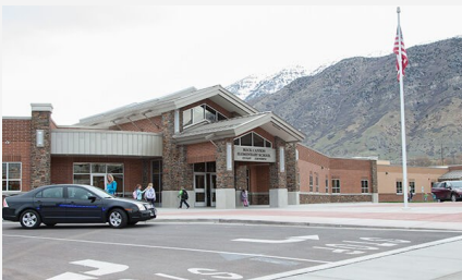
Rock Canyon Elementary (K-6) Principal: Seth Hansen Enrollment: 515 Year Rebuilt: 2016
