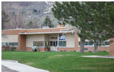
Wasatch Elementary (K-6) Principal: Chris Fuhriman Enrollment: 650 Year Built: 1949 Municipal Authority Bonds Ap- proved to rebuild November 2021
