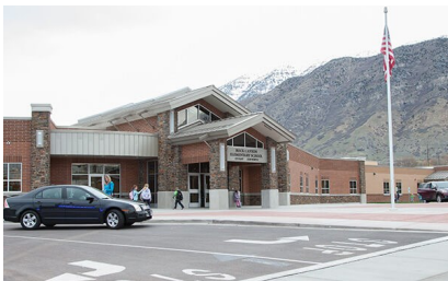
Rock Canyon Elementary (K-6) Principal: Seth Hansen Enrollment: 527 Year Rebuilt: 2016
