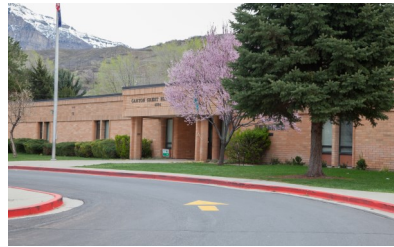
Canyon Crest Elementary (K-6) Principal: Sean Edwards Enrollment: 454 Year Built: 1982
