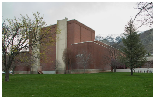
Timpview High School (9-12) Principal: Momilani Tu'ua Enrollment: 2,400 Year Built: 1974 Parital rebuild to be completed in 2024
