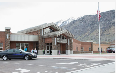
Rock Canyon Elementary (K-6) Principal: Seth Hansen Enrollment: 515 Year Rebuilt: 2016
