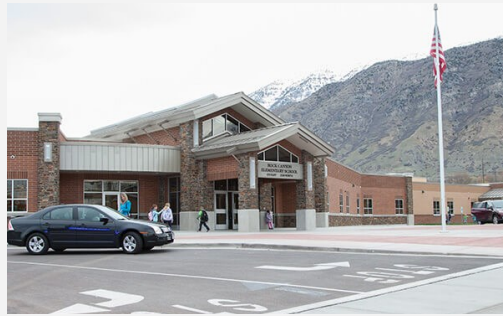
Rock Canyon Elementary (K-6) Principal: Seth Hansen Enrollment: 589 Year Rebuilt: 2016
