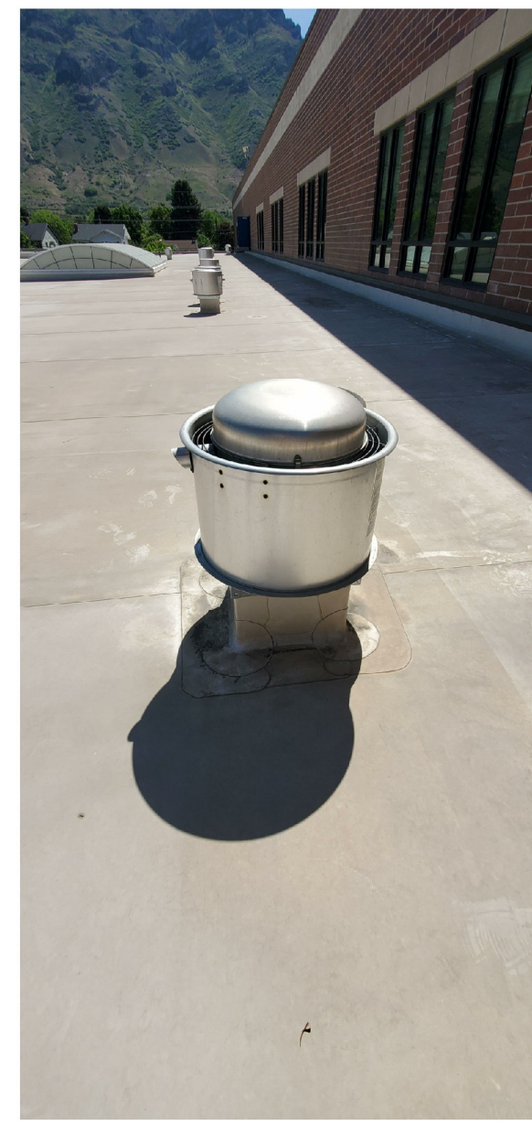
B4 TYPICAL ROOF FAN 4 A007 | SCALE: 3/4" = 1'-0"
