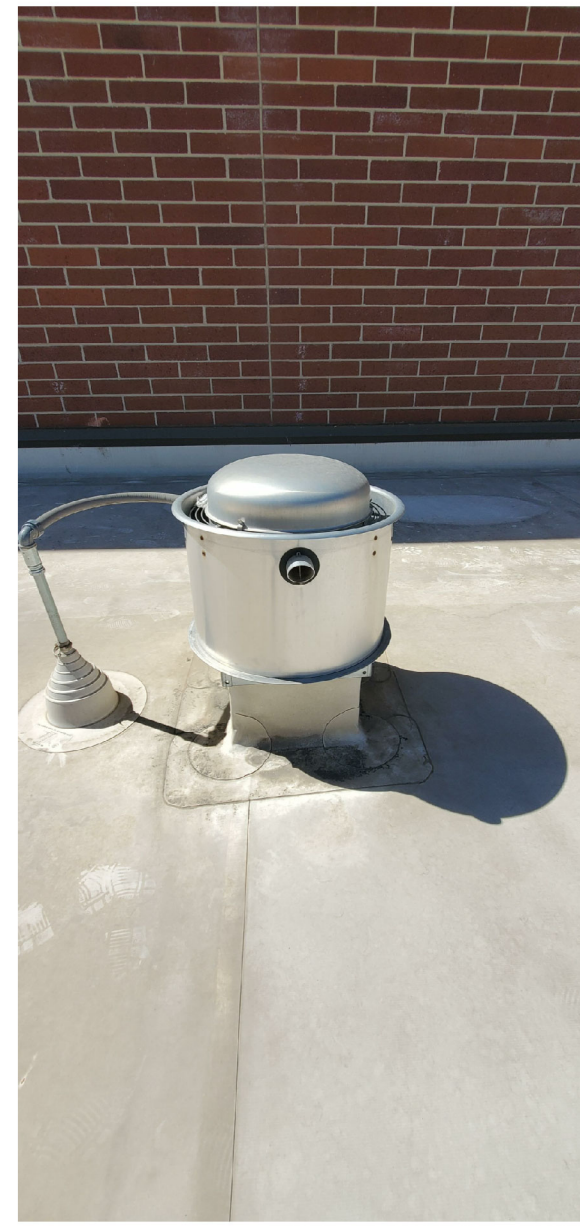
B3 TYPICAL ROOF FAN 3 A007 | SCALE: 3/4" = 1'-0"
