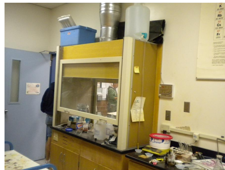
Figure 21. Science Room Fume Hood
