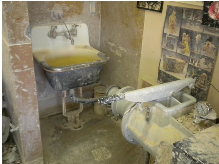
Figure 27. Pottery Area Sink and Clay Trap
