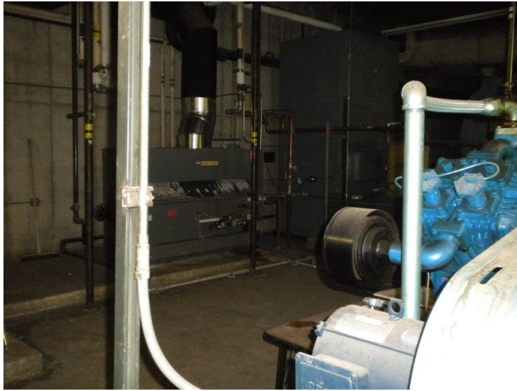
Figure 35. Laars Domestic Water Heater
