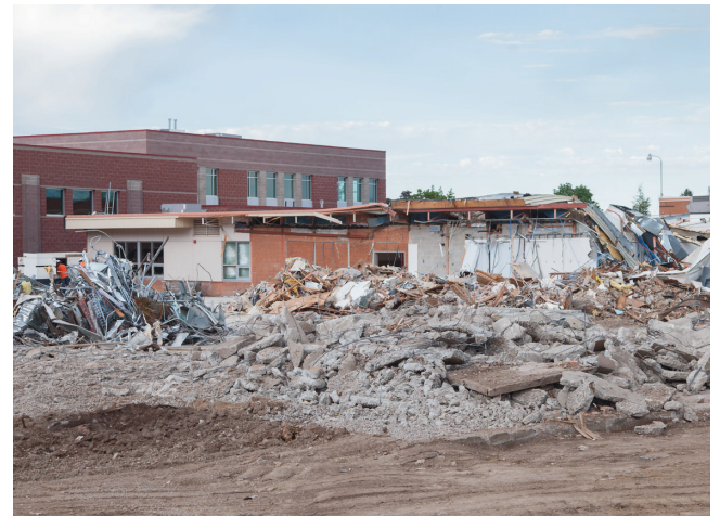
Photo of the old Edgemont building coming down on June 21, 2017
