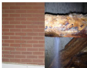
Cracked Exterior Brick Wall and Mortar Corroded Downspout Pipe Lines
