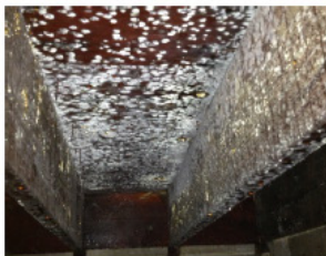
Moisture Damage to Floor Structure
