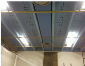
Heavy Concrete Roof on Unreinforced Masonry Walls
