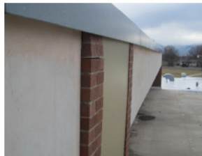
Cracked Exterior Brick Wall and Mortar
