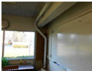
Exposed Plumbing Pipes Impact Learning Space
