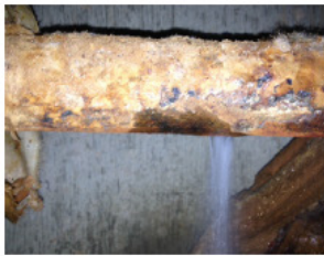
Corroded Steam Pipe Lines
