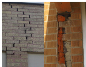
Cracked Exterior Brick Walls and Mortar, Crumbling Brick at Structural Beam
