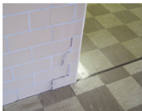
Cracked Interior Brick Walls and Mortar
