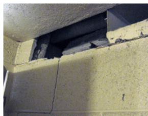
Cracked Structural Block Walls and Mortar, and Falling Wall to Roof Connection
