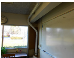
Exposed Plumbing Pipes Impact Learning Space
