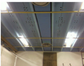
Heavy Concrete Roof on Unreinforced Masonry Walls
