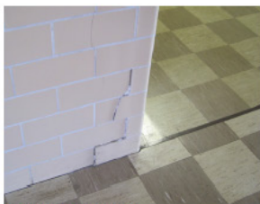
Cracked Interior Brick Walls and Mortar
