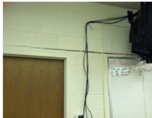
Cracked Interior Brick Walls and Mortar
