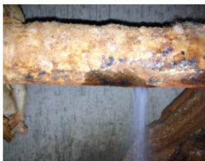
Corroded Steel Beam Pipe Lines
