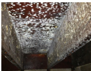
Moisture Damage to Floor Structure
