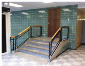
Non Code-Compliant Guardrail and Handrails
