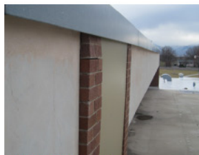
Cracked Exterior Brick Wall and Mortar
